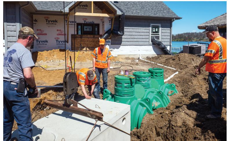
After effluent is treated by the Norweco Singular system, it passes to a concrete dosing tank being set in place by Dave Flory (left), James Sanders, Josh Sanders, and Dervin Witmer.
