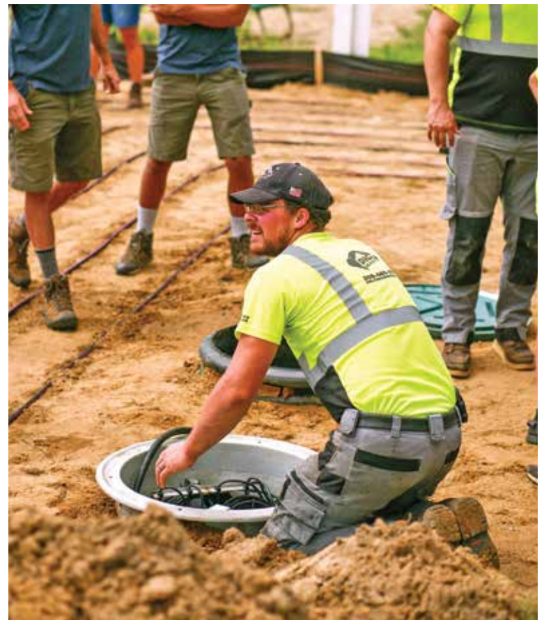
▼ James Sanders from Dig-It Excavating lowers the SludgeHammer unit into place during the educational outing at the Paw Paw job.
